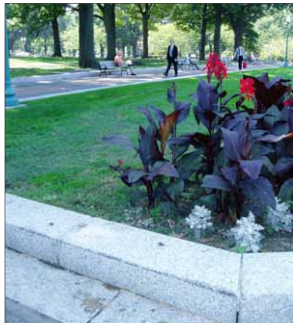
Curbed planting beds retain mulch and plant material, as well as discourage pedestrian traffic.
