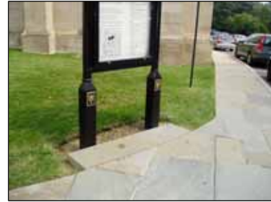
Hard platforms for seating, trash receptacles, and signs reduce use impacts on turf.
