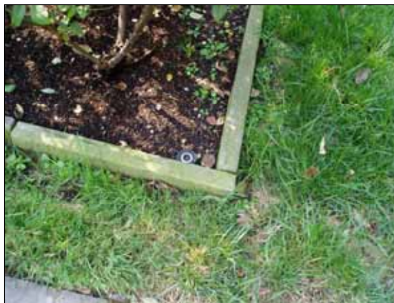
Planting bed edged to protect irrigation head and retain soil.
