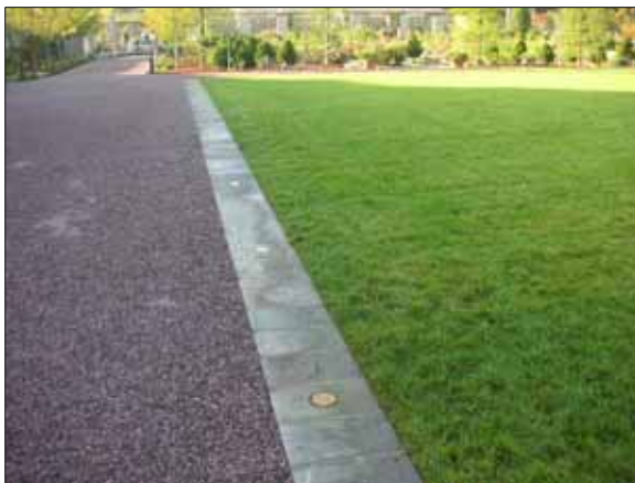
Stone edge containing built-in tent anchors.
